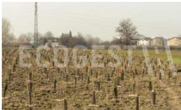
Naturalistic engineering works
