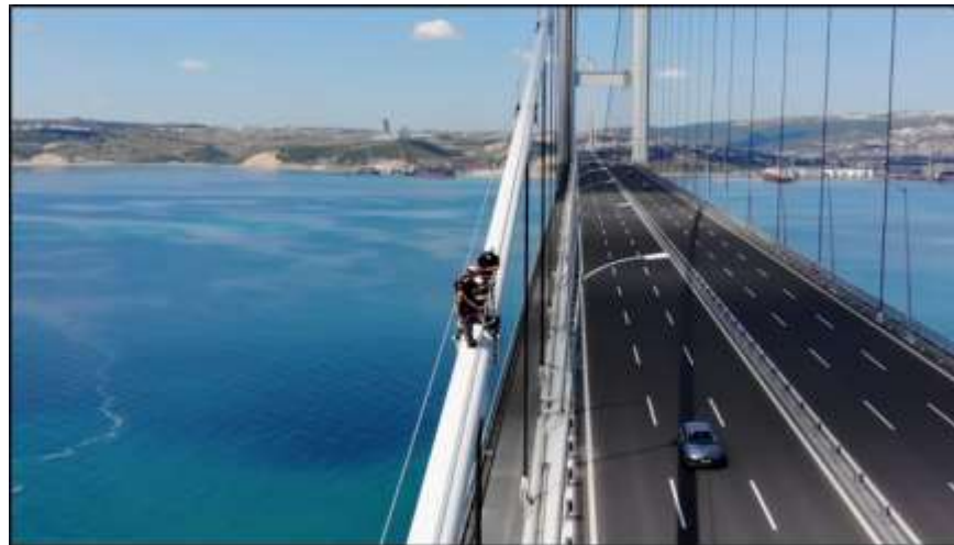
Elongation measurements of main cable clamp rods
