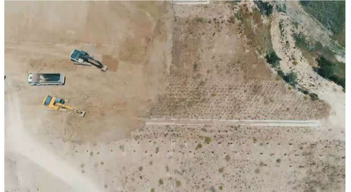
Earthworks working progress monitoring
