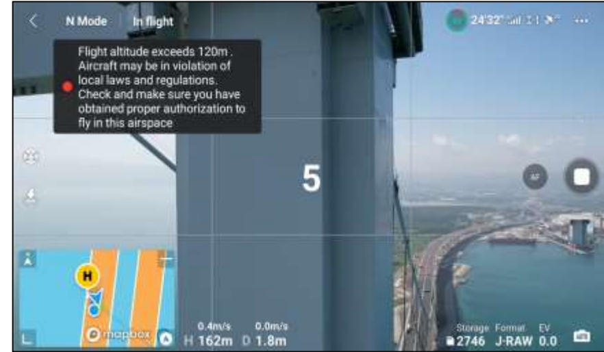
Main rope inspection
