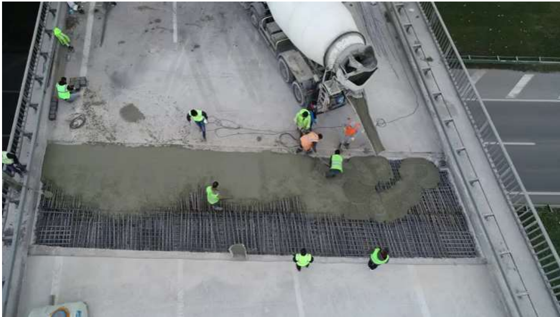
Monitoring of Maintenance Works
