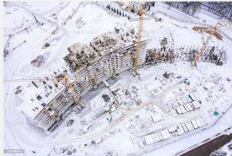
Identify high-risk days to increase safety on construction site
