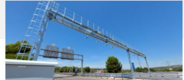
2 dual gantries Non-stop 120 km/h Without barrier
