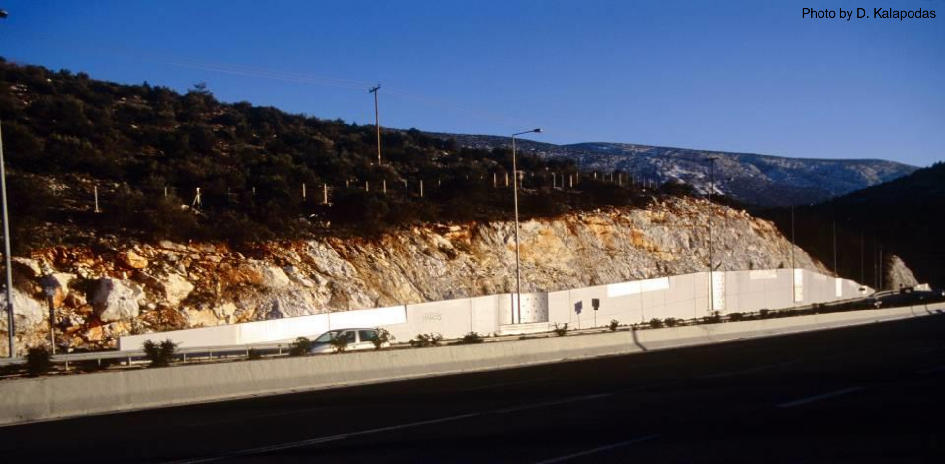
Concrete rock-trapping walls of variable height following the mountain cut skyline
