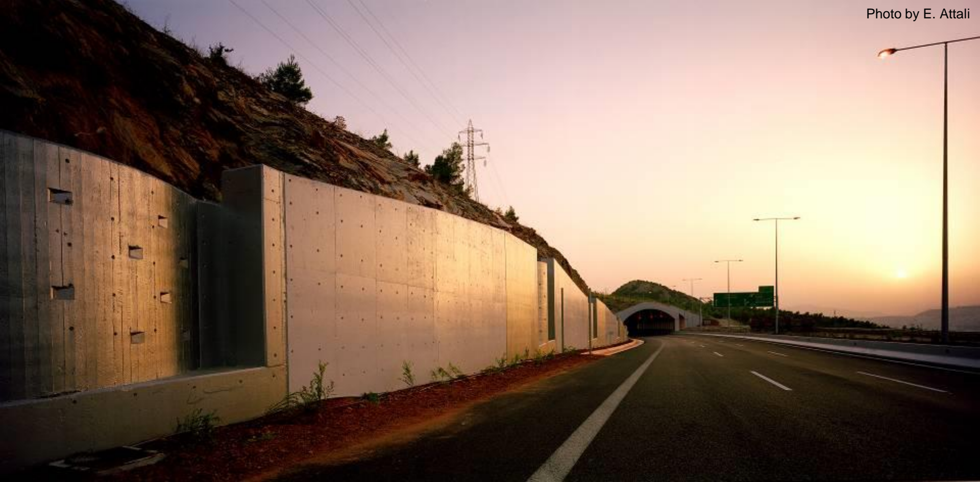
Concrete rock-trapping walls painted in silver and light gray, reflecting the sky color
