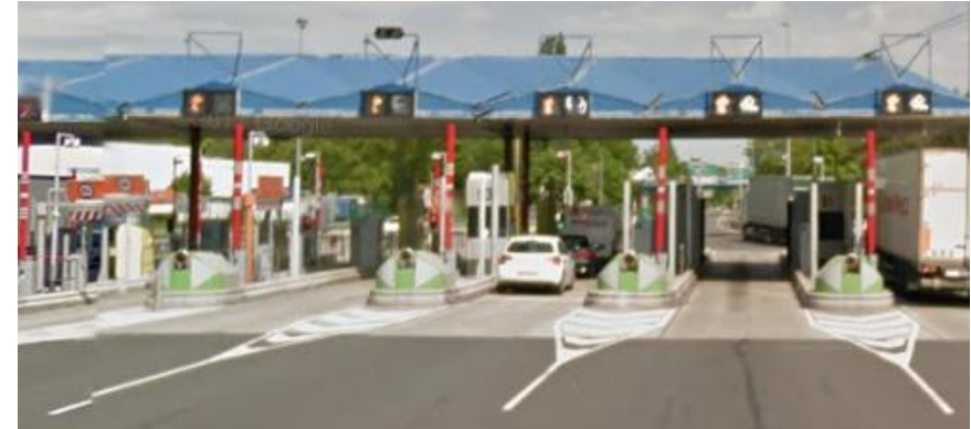
Toll plaza situation
